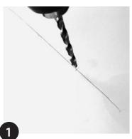
Check product orientation. Mark hole positions from brackets pre installed on MOMO-L Power base (2 per metre/40") and drill if required.
